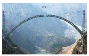
deep gorge, and the main arch has a span length of 467 metres, which Indian Railways claims is the largest in the country. Once the arch is complete, viaduct and track laying work will start, learns TOI
